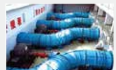
Drainage & Wastewater treatment
